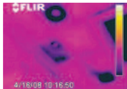
A leaking sprinkler head in a newly-built home
